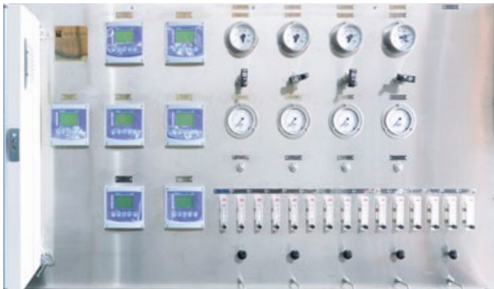
One of several water sampling panels utilizing Thornton M300 transmitters to monitor pH, conductivity and dissolved oxygen levels in a Thailand natural gas-fired power plant. This panel (partially shown) monitors two of the plant's six boilers.
